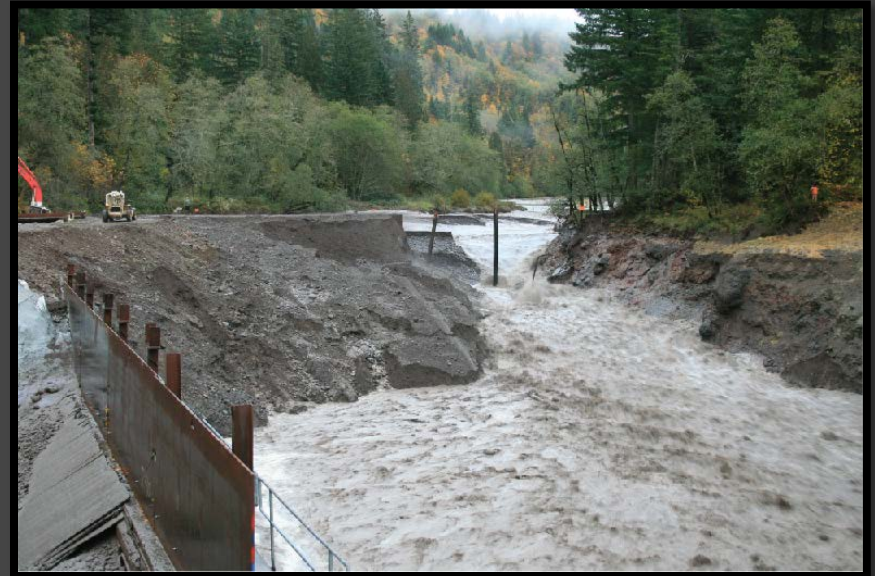
Marmot Dam removal Photo credit: USGS Cascades Volcano Observatory
